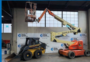
Skid Steer and Boom Lift
